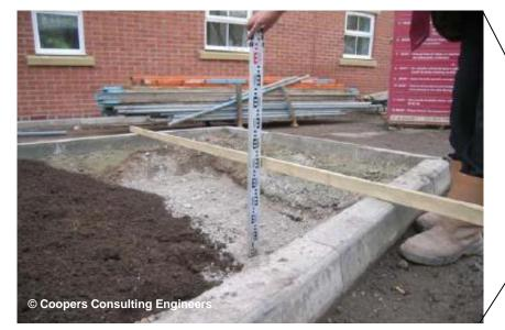
Photograph 1: Depth check of inert cover within area of public open space. Physical break layer and topsoil visible.
