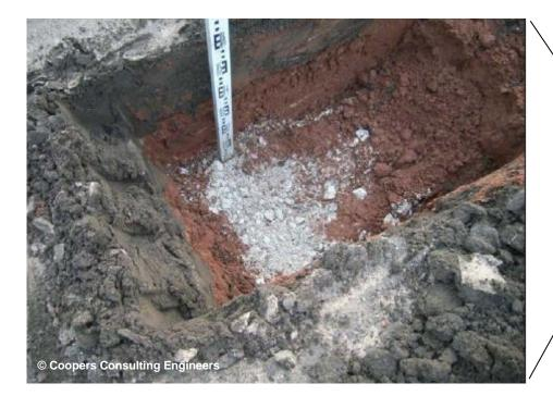
Photograph 8: Excavation within public open space and verification pit showing the presence of a remediation break layer at the base, a crushed sandstone inert fill overlain by topsoil.
