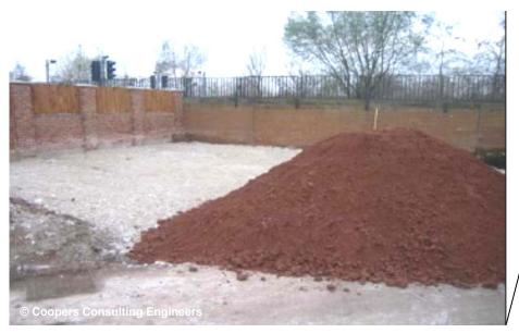
Photographs 9 and 10: Inert crushed sandstone being delivered with remediation break layer visible in Photograph 10. The spatial area of the remediation can be observed from these photographs (old terrace housing in Photograph 9 and traffic lights in photograph 10).
