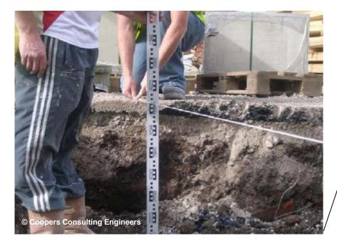
Photographs 5 and 6: Depth check of inert cover within rear gardens. Taut string line spans across excavation.
