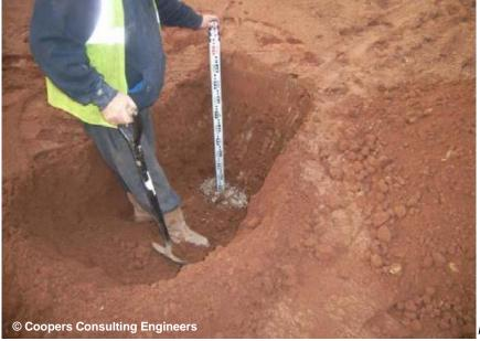
Photographs 11 and 12 show the remediation of the rear garden, with a significant depth (1.0m) of inert cover.
